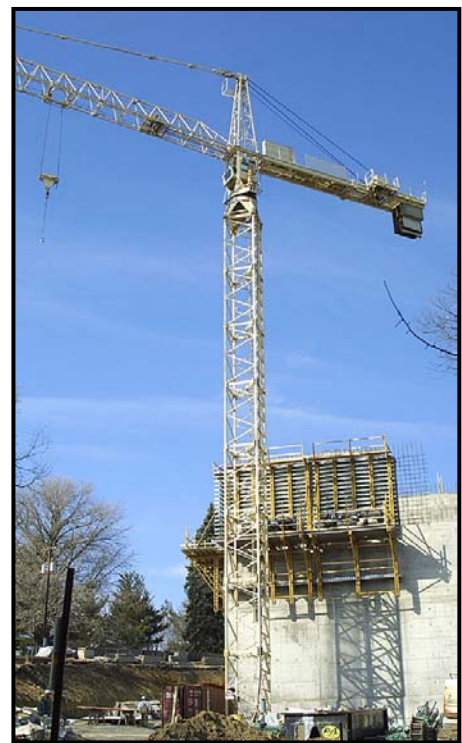
Photo 1 -- Hammerhead crane at site.
