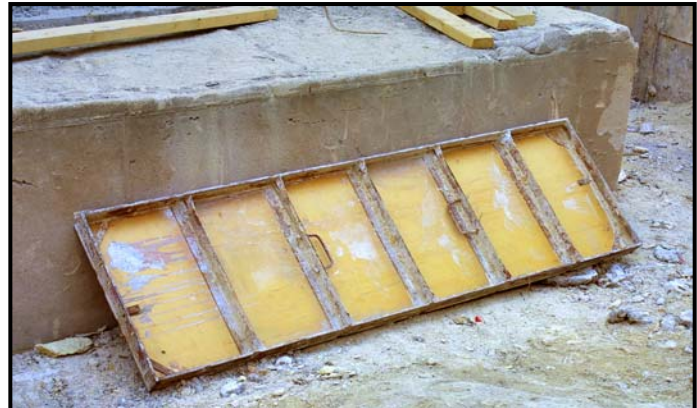
Photo 3 -- Typical plywood and steel cement form.
