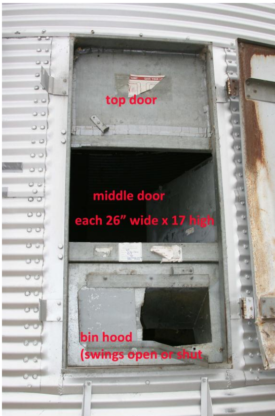
Exhibit 2. Side access door
