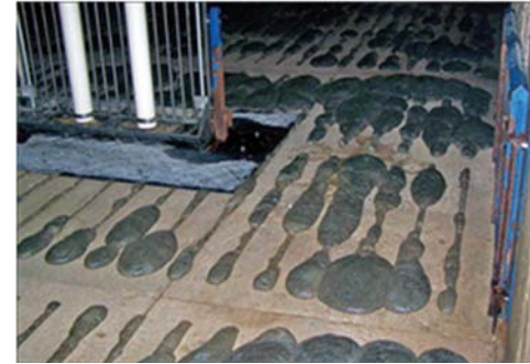
Foaming pit coming through floor slats (from University of Minnesota, http://www.extension.umn.edu/agriculture/manure-management-and-air-quality/feedlots-and-manure-storage/foaming-manure/ )
