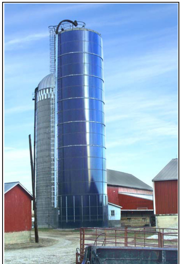
Photo 2 – Outside view of silos showing the attached shed and adjoining feedlot.
